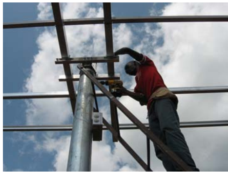
Installing Rack for Panels
