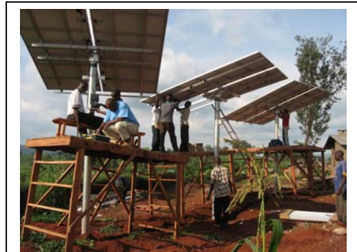
Erecting Pole Mounted Panels
