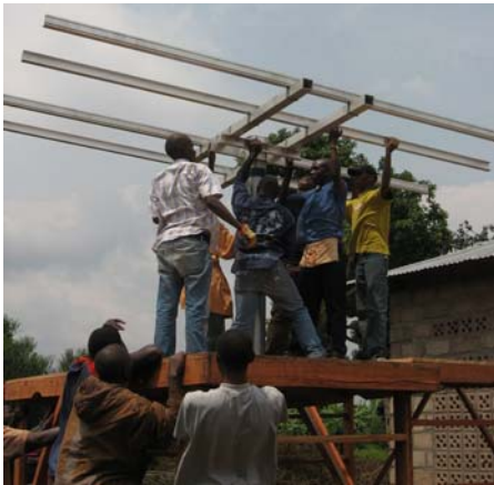
Installing the Rack on the Pole
