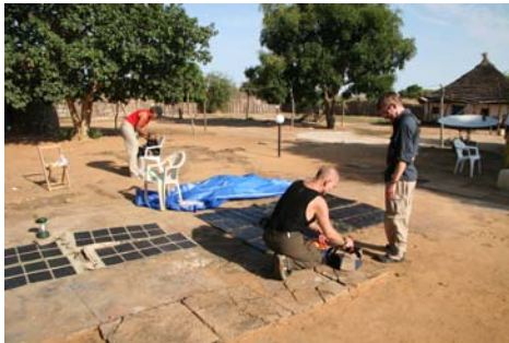
Walt, setting up solar equipment
